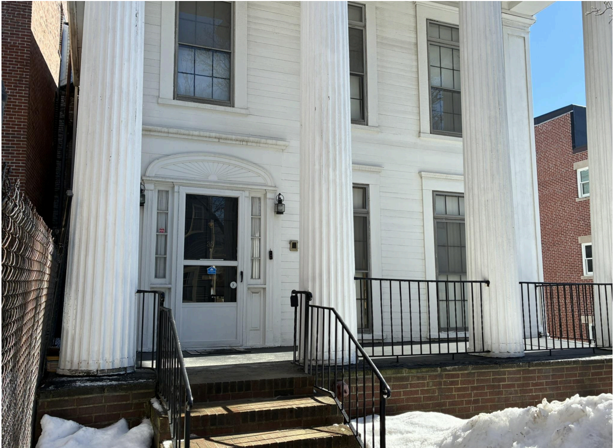
Figure 8. Detail of the front entrance of the Swallow Mansion (March 4, 2026).
